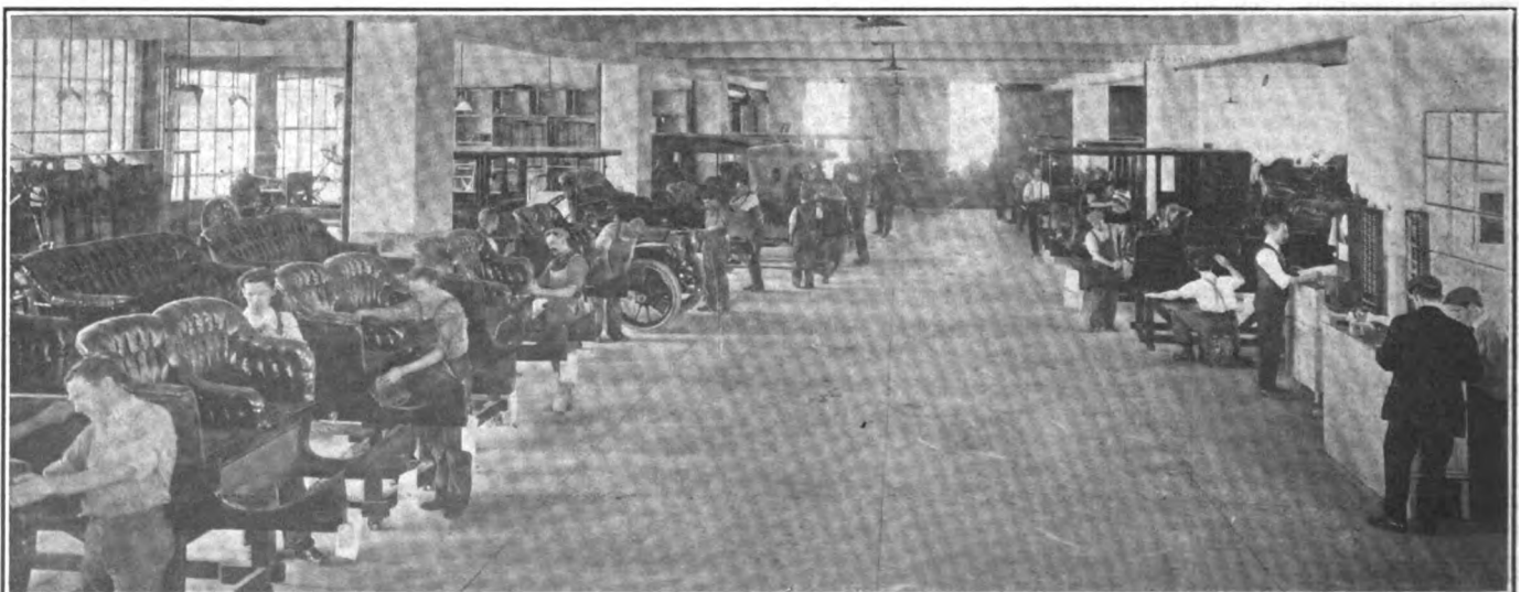
Fig. 3—A portion of the body painting department on the fifth floor. Job costs for this department are made up at the right
